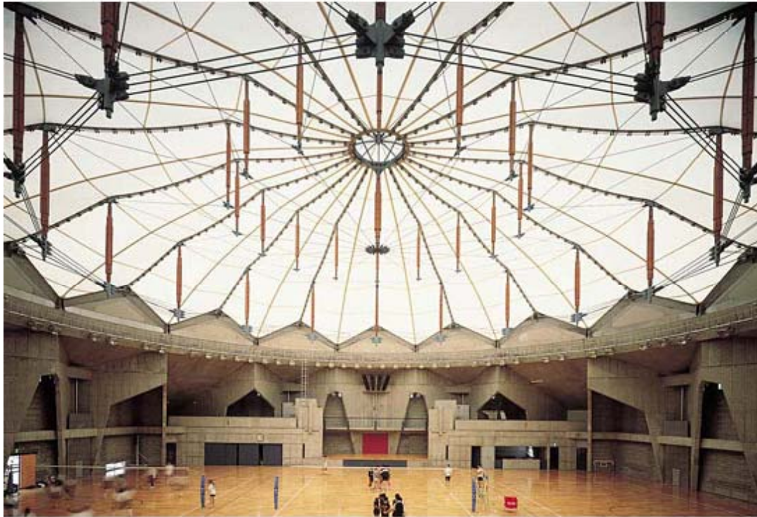
Kano Dome (1991, Shizuoka, Japan)
